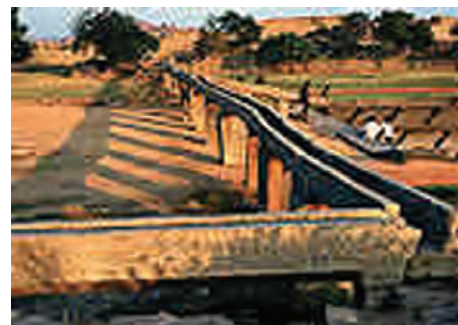
Fig. 7.5 An aqueduct leading into the royal centre
