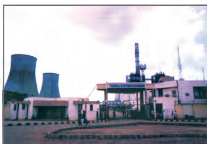
Fig 3.10: A view of a Thermal Power Station
