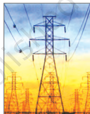
Fig. 3.7: National Power Grid to supply Electricity
